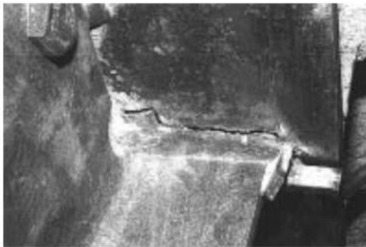
a. Fracture at Fused Zone
